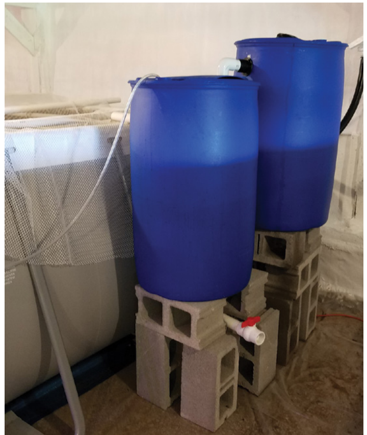
Figure 5. A simple settling chamber and a biofilter. The settling chamber is higher to allow water to travel to the biofilter via gravity. The filters are supported by concrete blocks. Note the protected surfaces in the room and covered tank.
