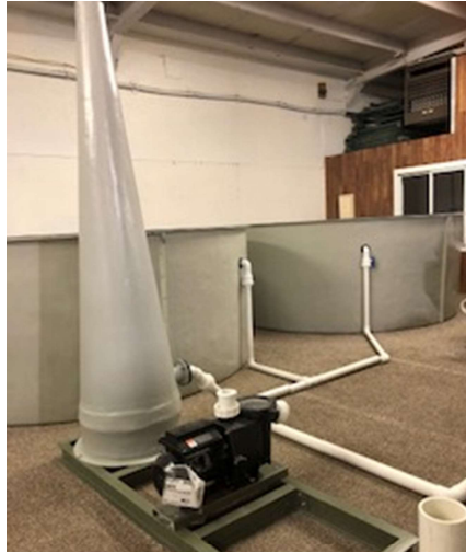
4 - 10' diameter fiberglass tanks Skidded Oxygen Saturator / Sparus Pump DO monitoring
