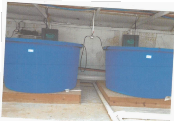
1200 gallon, 8' diameter, Poly tank, round
