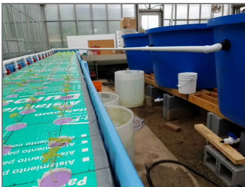
Figure 4. System setup with 250 gallon tanks, the side drains, and raceway with inlets delivering water to the plants. (Photo by Neal Kolonay)
