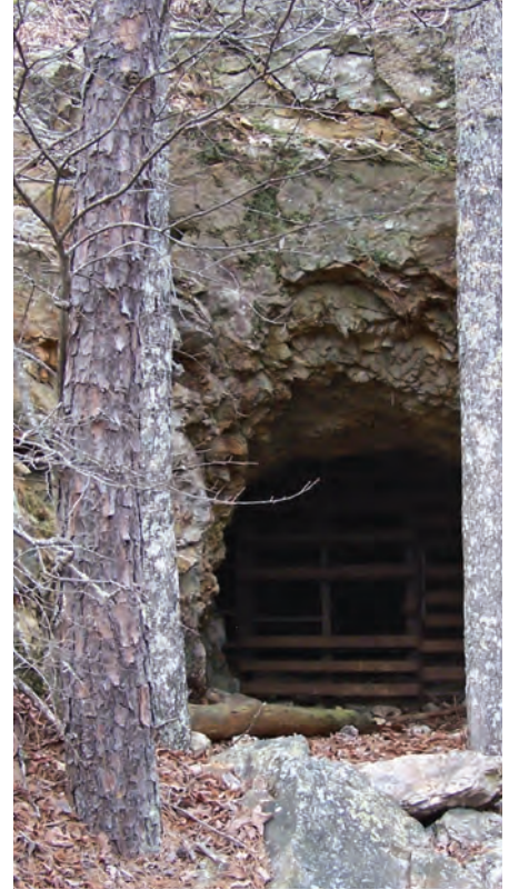
An abandoned mine gated for public safety and to protect hibernating bats.
